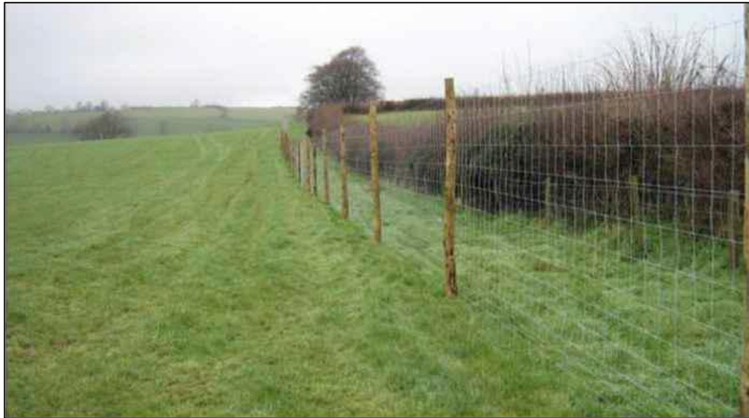
Plate 13 Typical Deer Fencing
