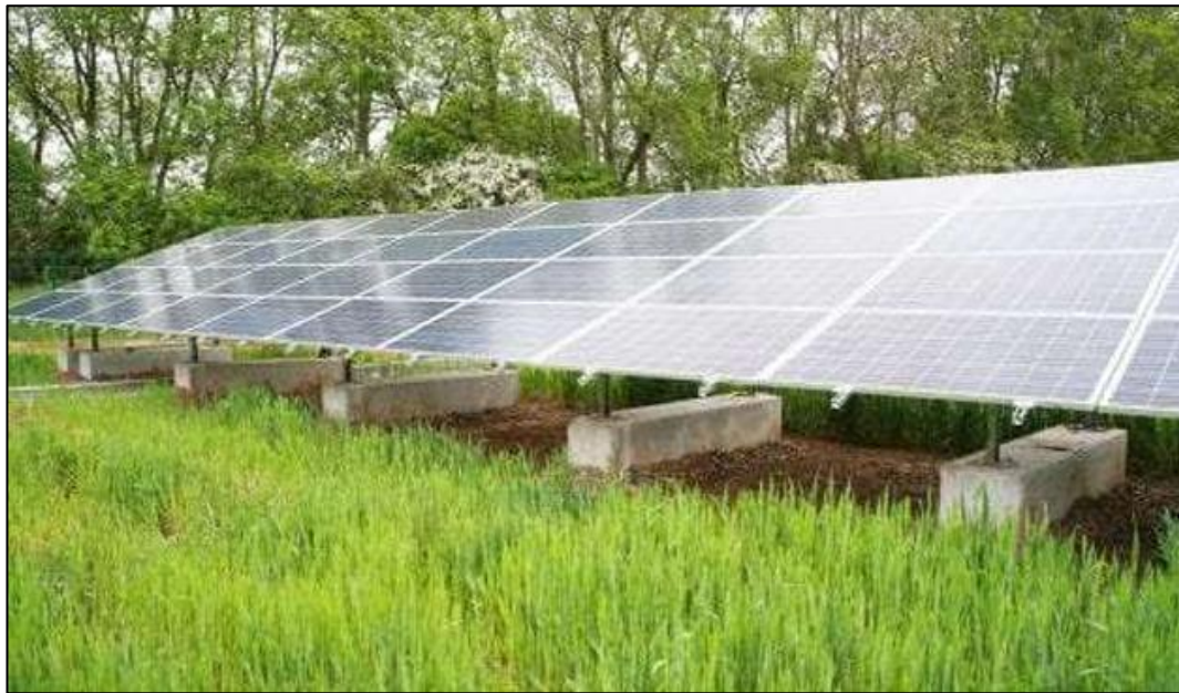
Plate 4 Fixed Panels on Concrete Feet
