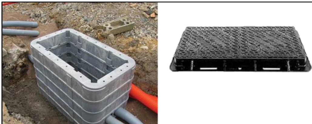
Plate 12 Fibre Chambers (construction and external appearance)
